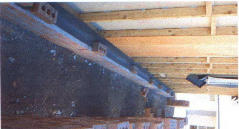
Brick Vent Flashing
